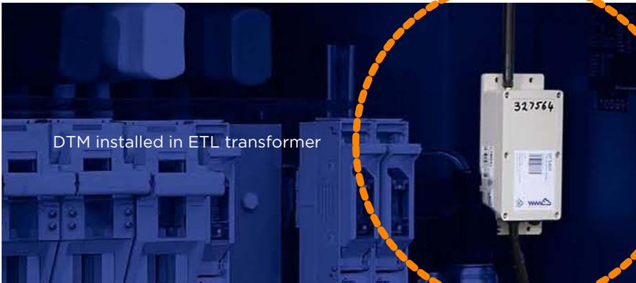
In its simplest form, the WMAAC DTM connected MDIs, providing 1/2 hourly current data so monthly, weekly and daily current demand is always available. The DTM also provides alarming for voltage loss and over-temperature of the transformer oil.
